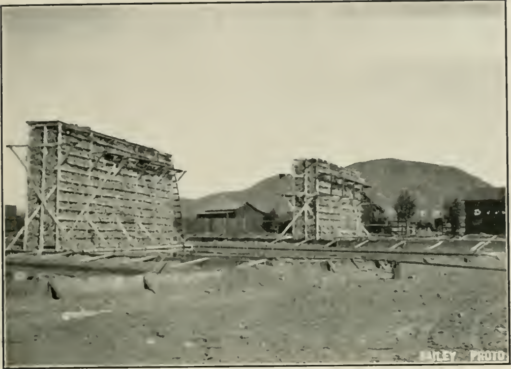
BRUSH RACKS FOR CRYSTALLIZING BORIC ACID ON—BARTLETT WORKS, DAGGETT, SAN BERNARDINO COUNTY.
